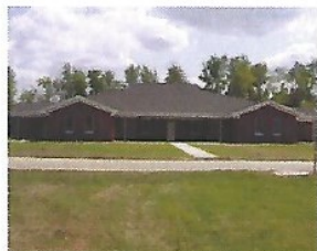
Fr. McGivney Hall Student Dormitory
